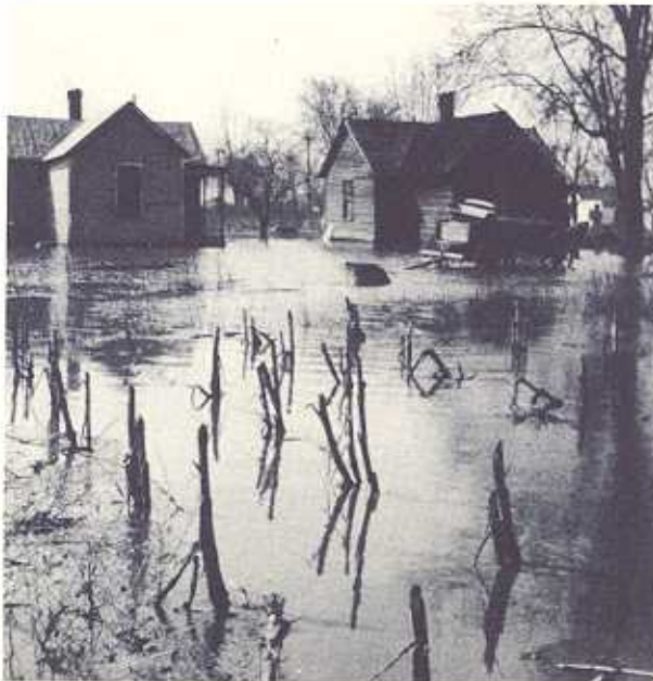
A situation that requires emergency action from the Sanitary Engineering Division
