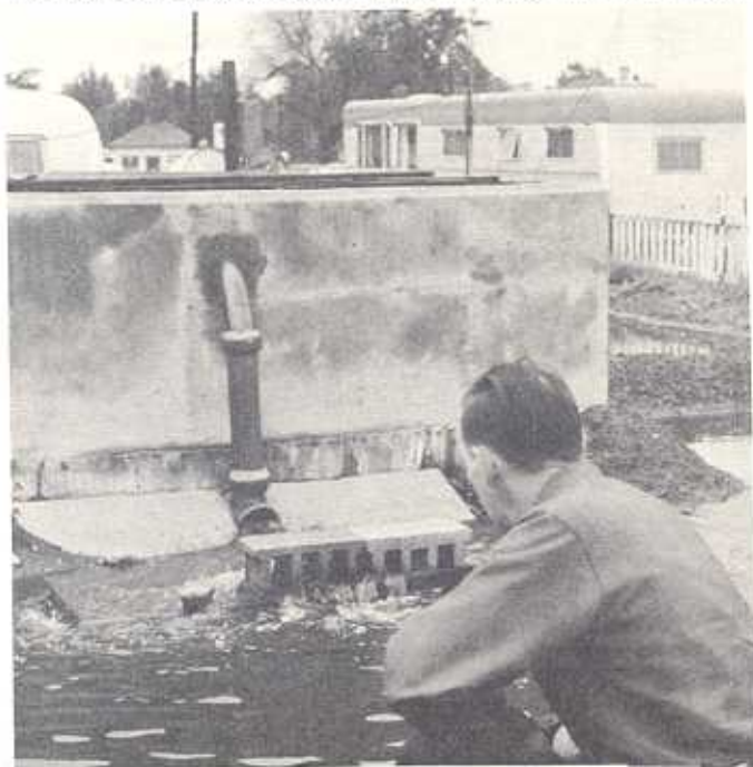
Observing operation of sewage treatment facilities at a trailer park.
