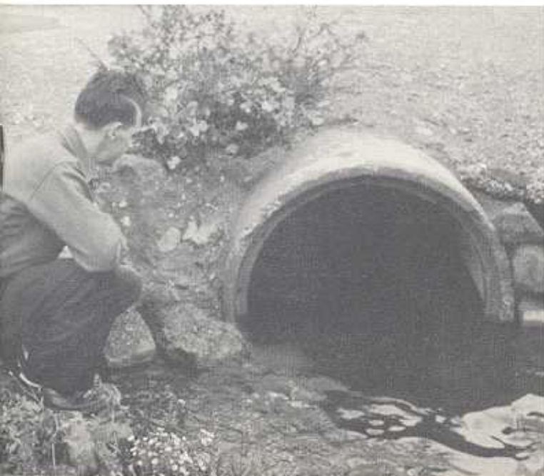
Checking storm sewer outlet for evidence of stream pollution.
