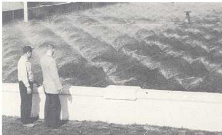
Observing operation of trickling filter at municipal sewage treatment works.
