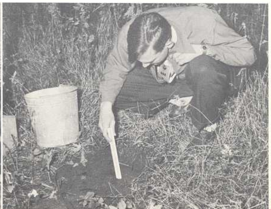
Running a percolation test to determine ability of soil to absorb sewage from private residence in area where public sanitary sewers are not available.
