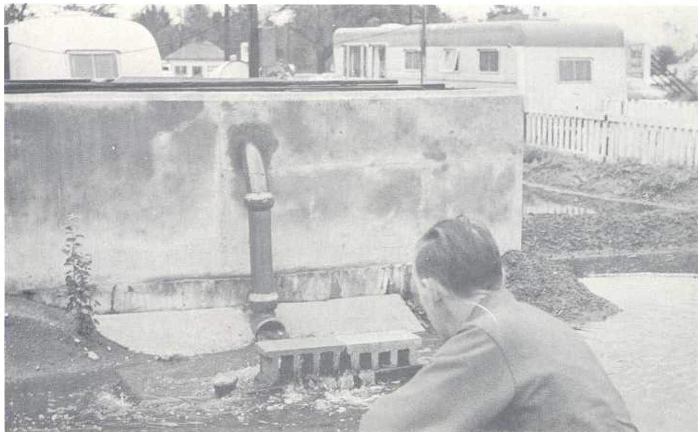
Observing operation of sewage treatment facilities at trailer park.
