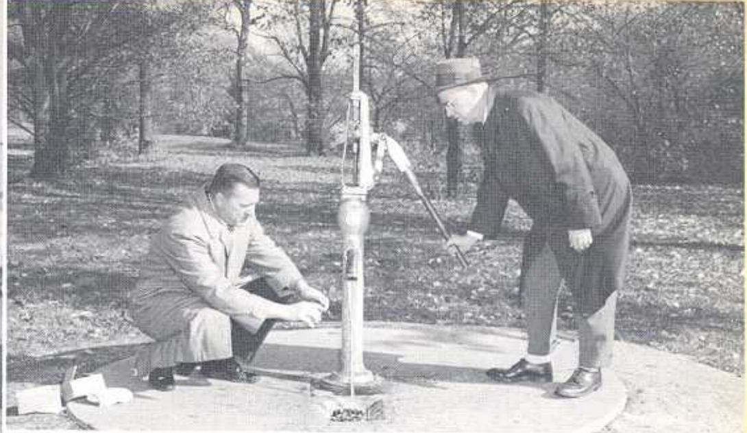
All wells in the Forest Preserve District are sampled for bacteriological safety every year and those wells not considered safe are taken out of service.
