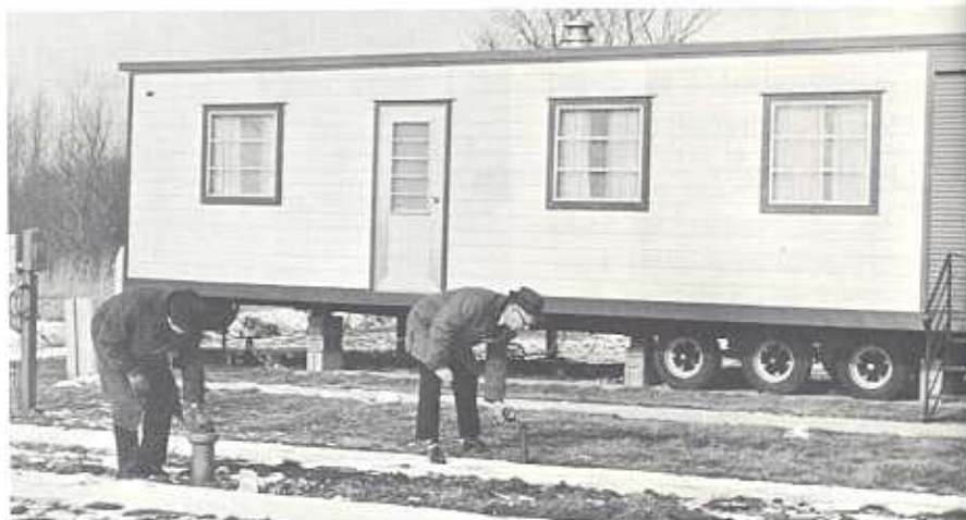
Trailer parks and motels are inspected and licensed to determine compliance with state and county codes.
