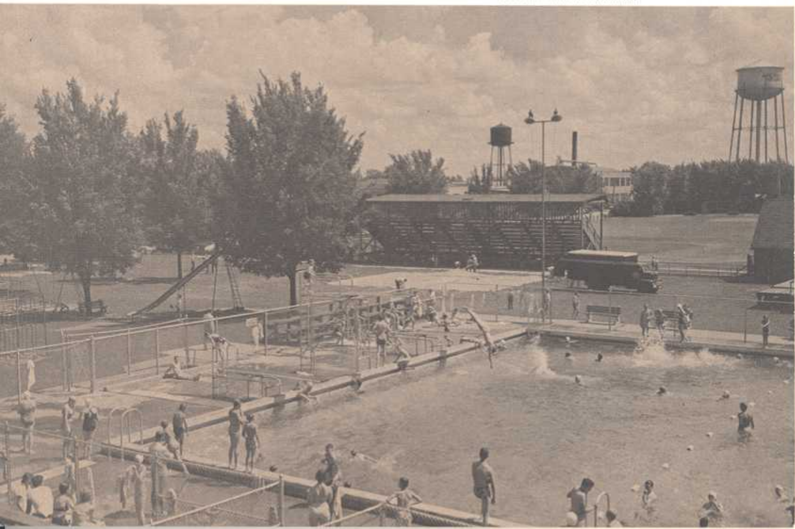
Public swimming pools both indoor and outdoor are inspected in order to ensure a healthful recreational environment.
