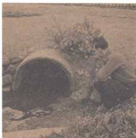
Field inspection of sewer discharging sanitary wastes to stream.
