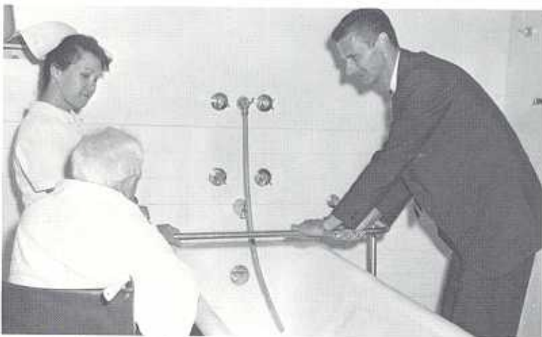
Installation check that the grab bar is safe and secure.
